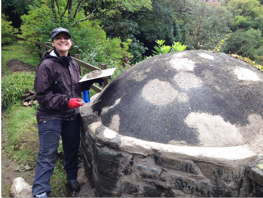
Dome at bridge entrance beautifully repointed!
